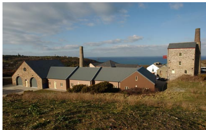
Formerly a derelict tin mine, Wheal Kitty has been transformed into high quality workshops
