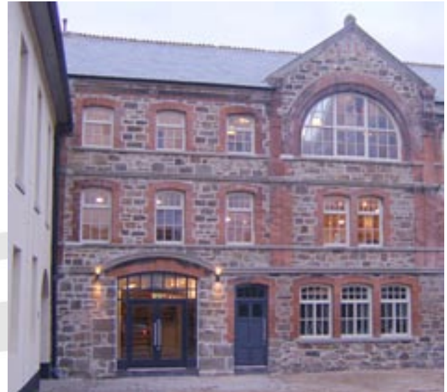
The refurbished White's Warehouse, part of Hayle Townscape Heritage Initiative
