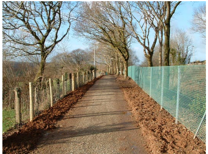
Part of the new Bodmin greenway, shortly after completion
